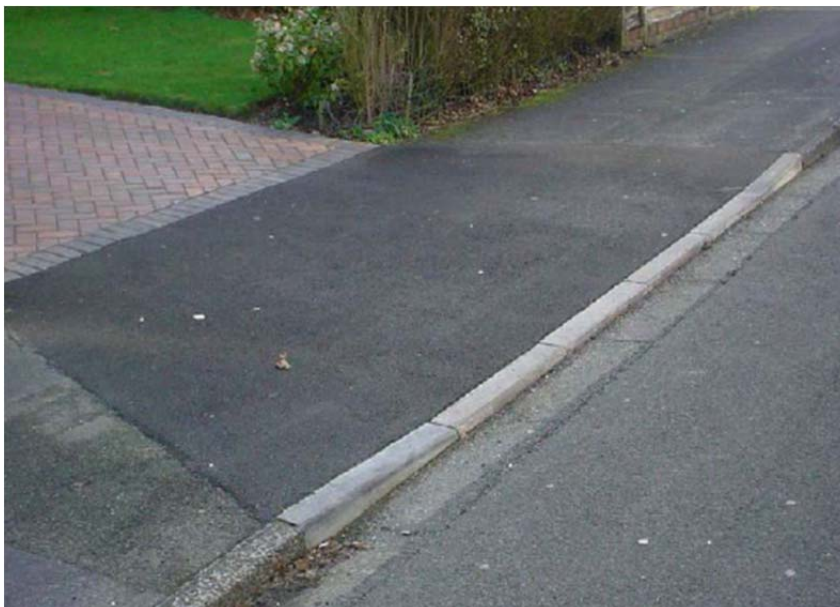
Figure 1. Typical Dropped Kerb
