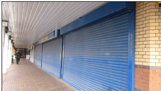
Photograph (left): Vacant Unit, Former Blockbuster Unit
