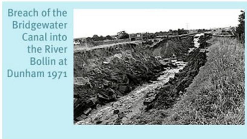
Figure 5-1: Bridgewater Canal Breach at Dunham
