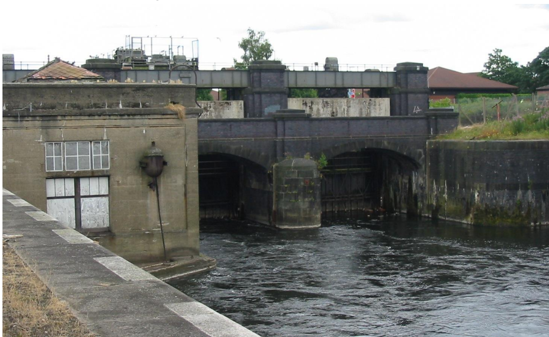
Figure 5-4: MSC Latchford Locks Sluice Gates
