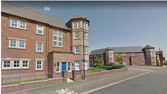
Existing buildings in Grappenhall Heys
