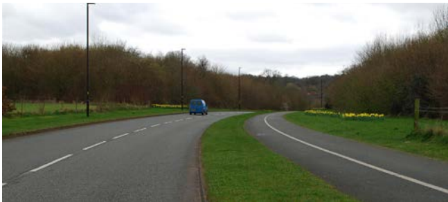
Existing view of Witherwin Avenue
