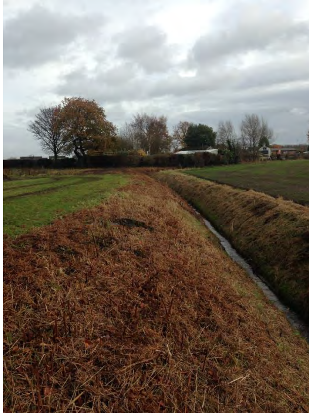
6 View looking southwards towards Willoways.
