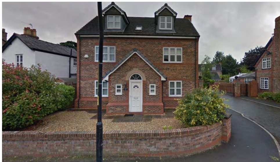
Fig 7.5 Examples of more recent development on the south side of Rushgreen Road, close to the site.
