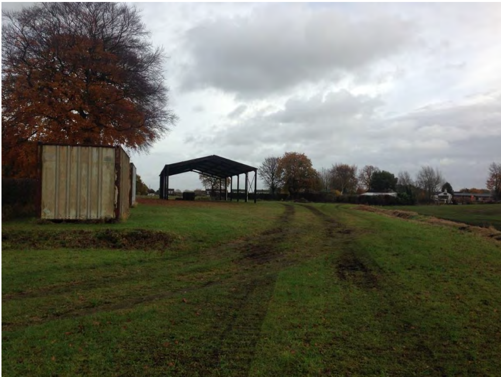
7. View looking eastwards towards existing agricultural buildings.
