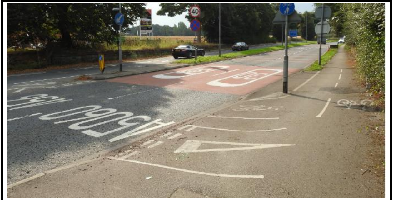
Cycle Lane on north side of Chester Road
