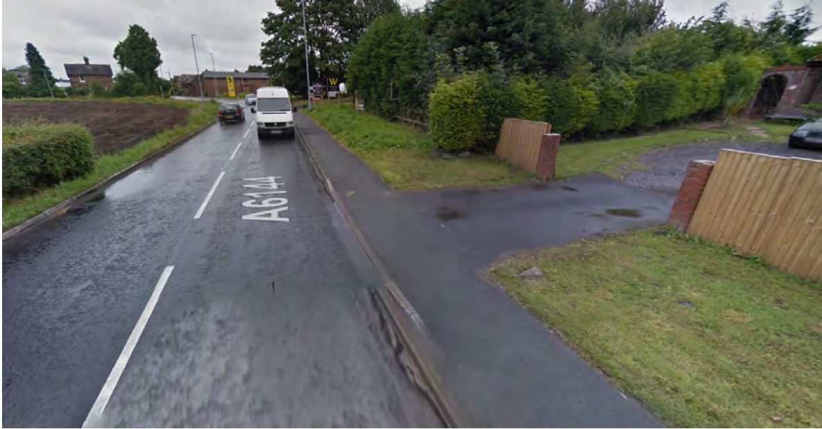
Approaching the site driving eastwards along Rushgreen Road.
