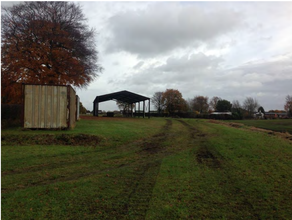
7. View looking eastwards towards existing agricultural buildings.
