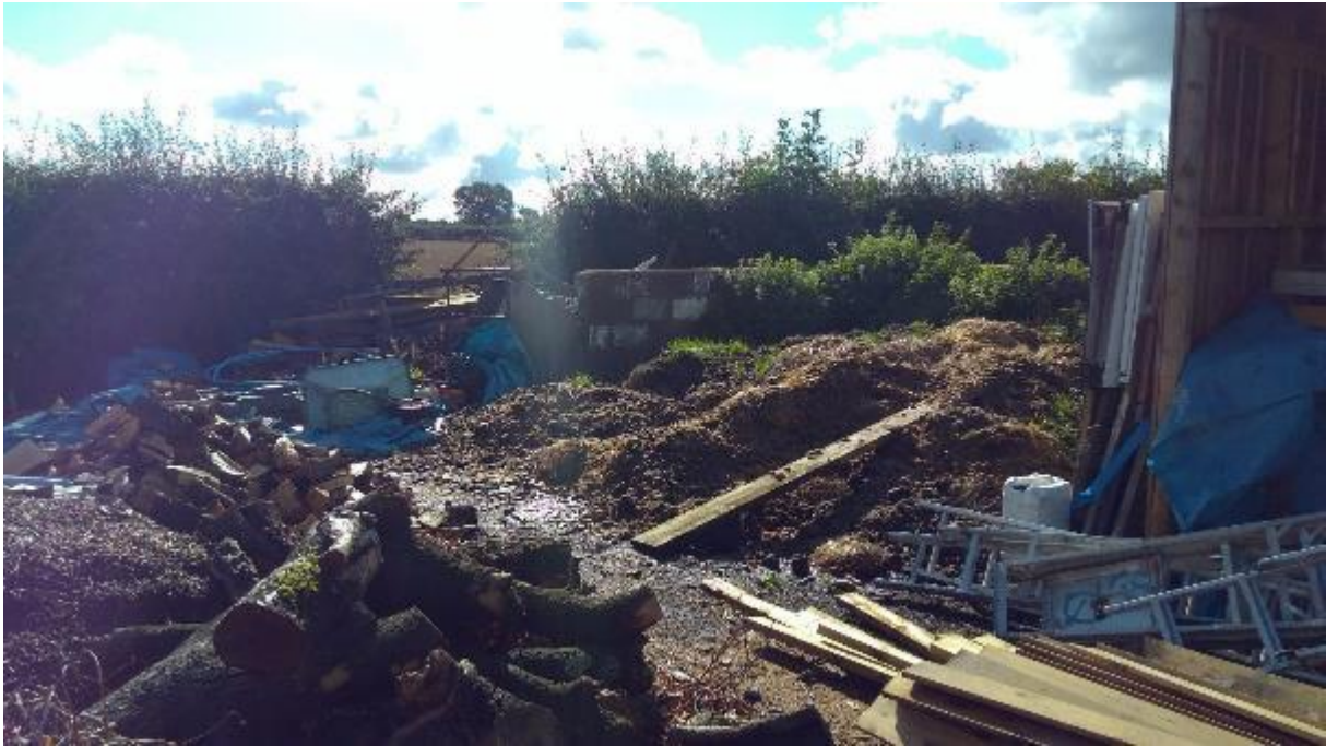
Photograph 12 – Manure stockpile in east of Site
