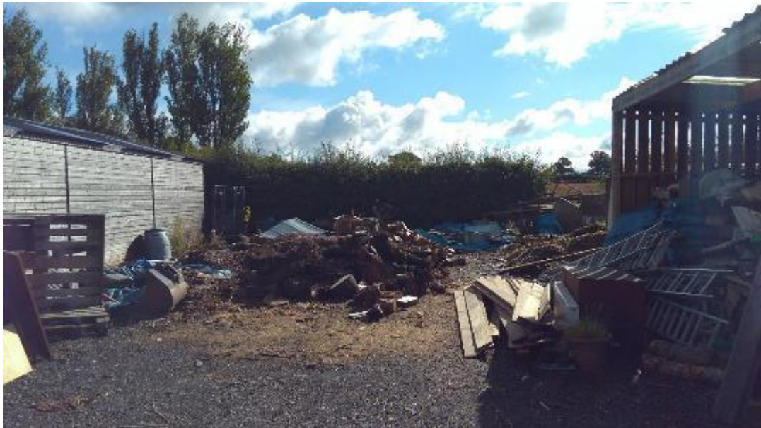
Photograph 4 – Stables, yard and lean-to in east of Site
