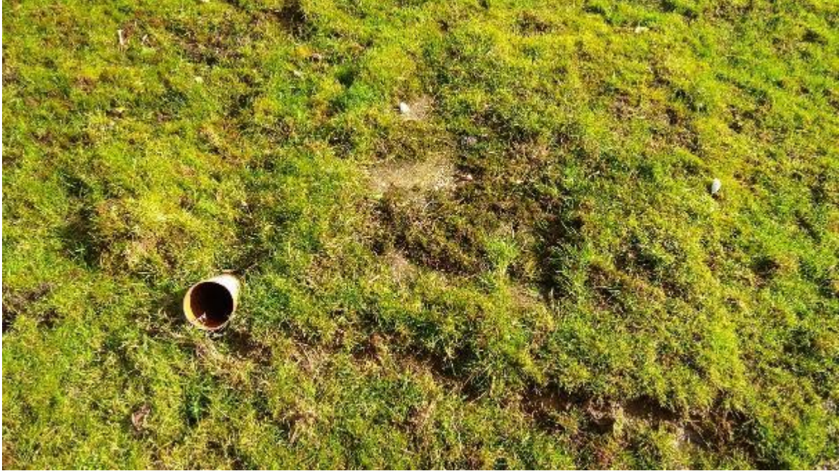
Photograph 5 – Land drain in southern corner of western field
