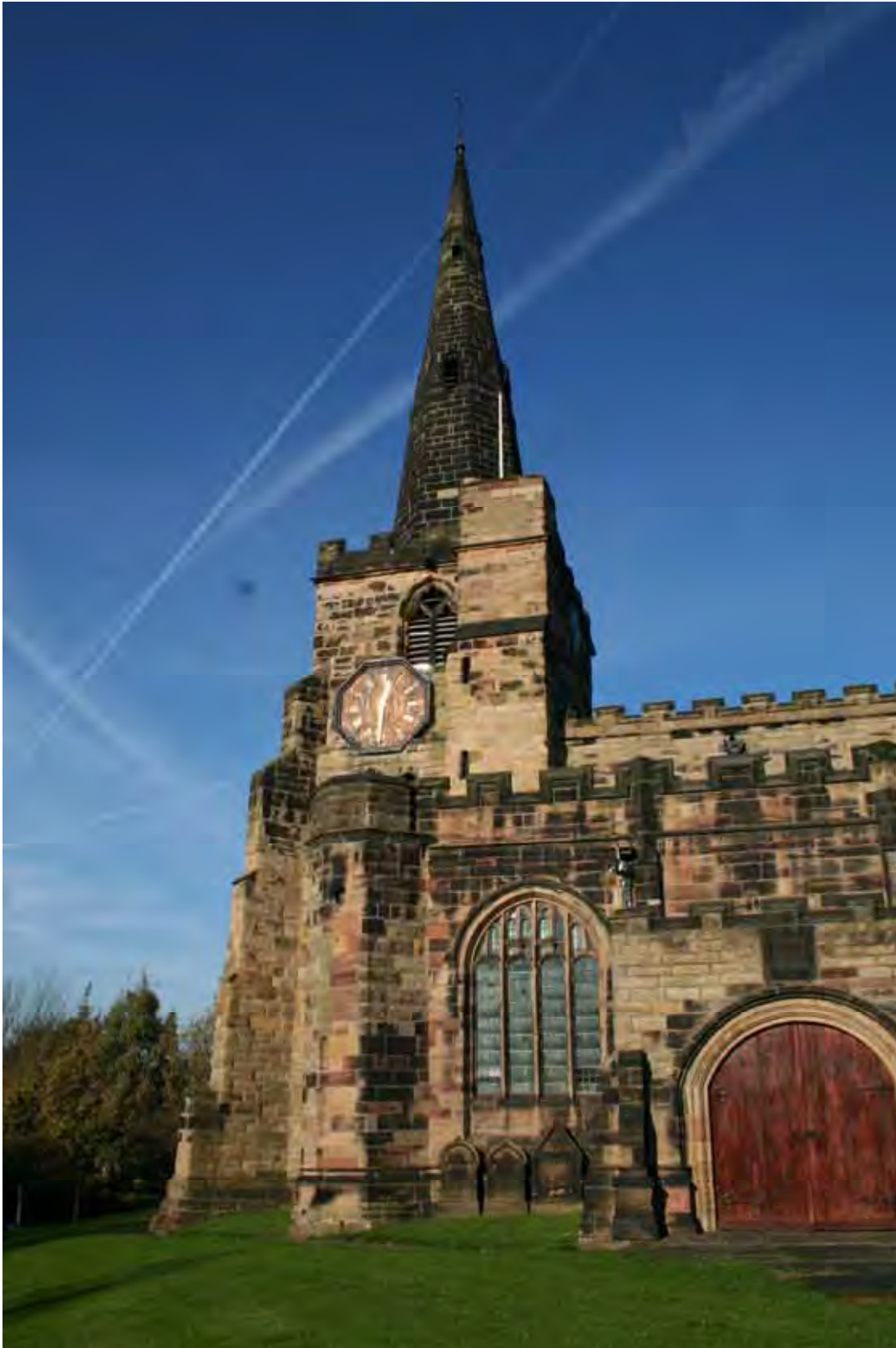
Photo 32a . South elevation of the historic Winwick Church - a very conspicuous landmark.
