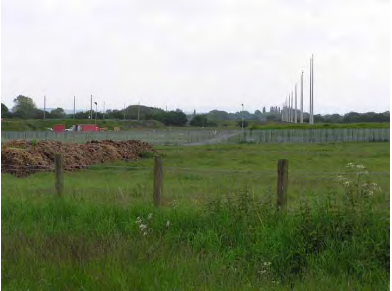
Photo 61a. Culcheth Carrs storage facility.
