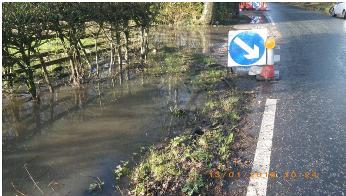
Figure 6: Image of flooding observed on 13 January 2016 to Stone Pit Lane.
