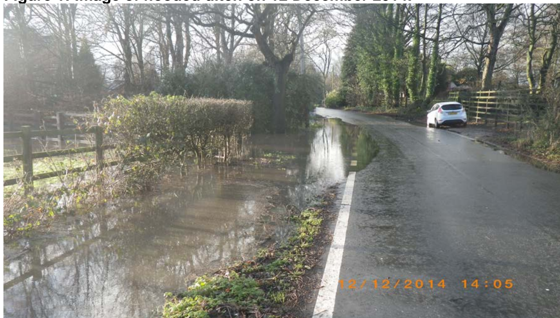
Figure 1: Image of flooded ditch on 12 December 2014.
