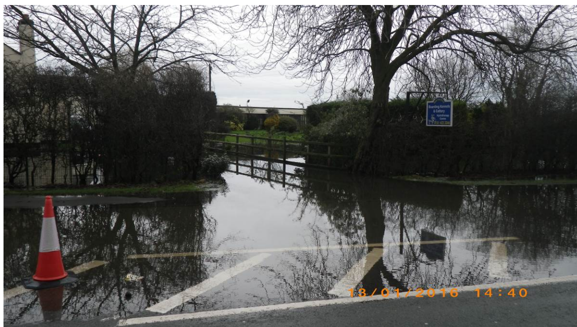
Figure 3: Image of Flooding to Entrance of Rose Tree Farm.
