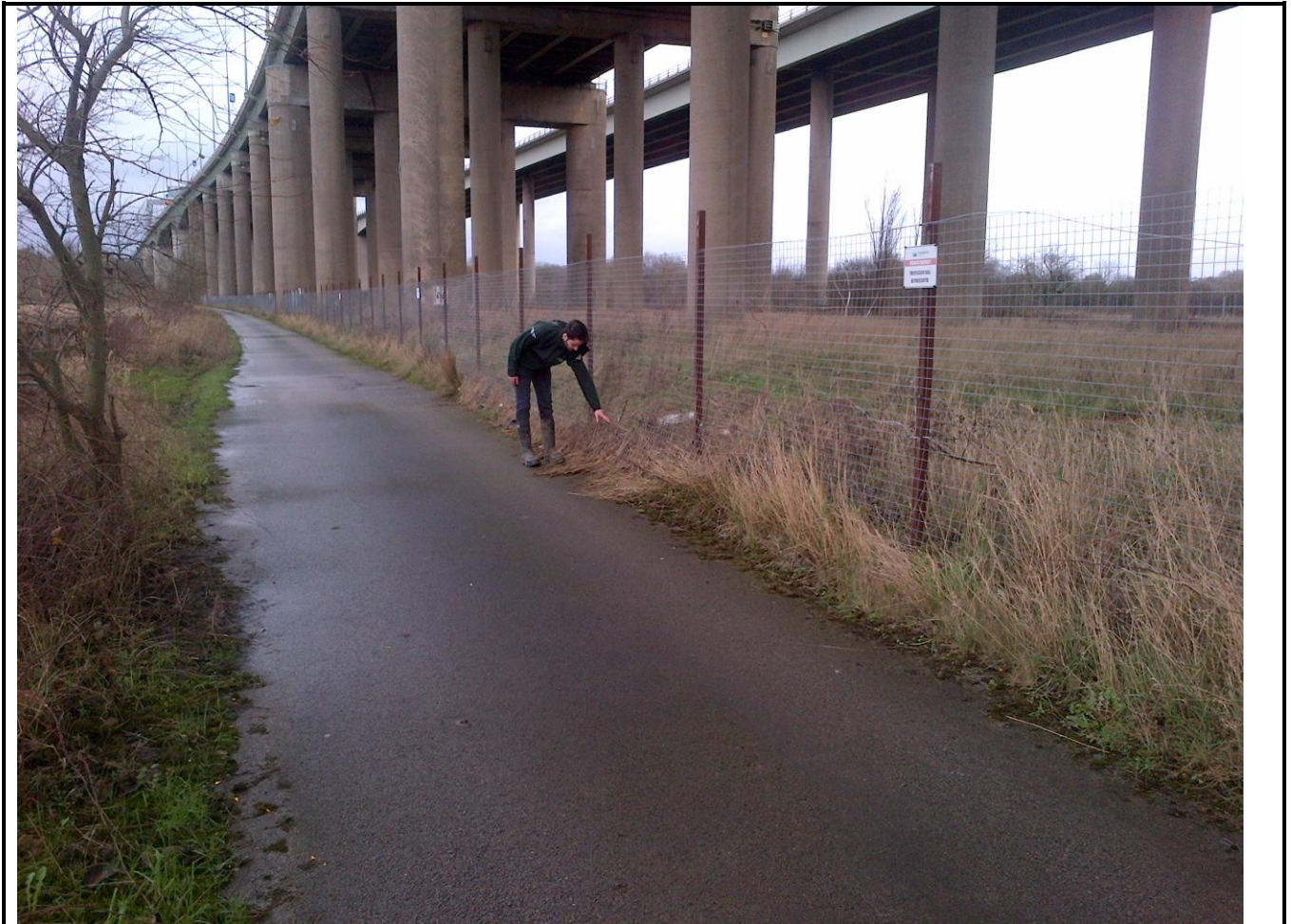
Photo 1. Flow under Motorway. From SJ6648487736, N. 27/01/16.
