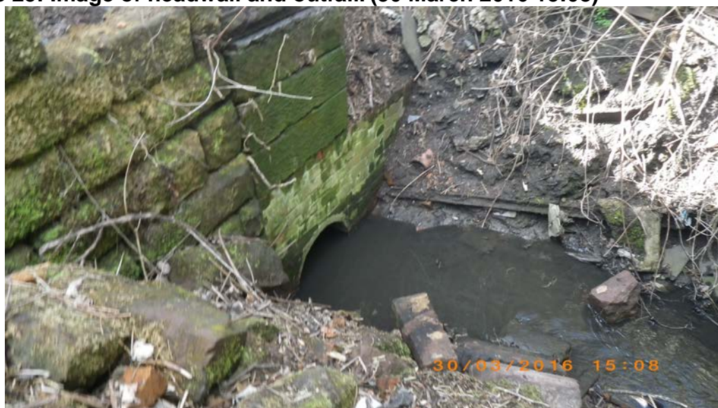
Figure 25: Image of headwall and outfall. (30 March 2016 15:08)
