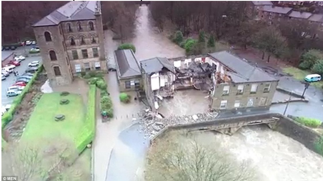
Figure 7: Image of the Waterside pub in Summerseat which collapsed on 26 December 2015 (Time Unknown) into the River Irwell.
