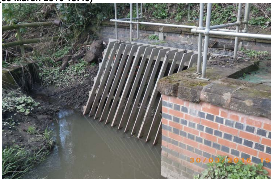
Figure 1: Trash Screen on Thelwall Brook at inlet to siphon under the River Mersey. (30 March 2016 15:40)
