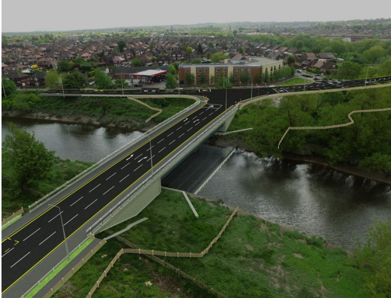
Figure 2: New bridge structure
