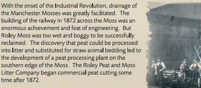
A two storey wood and corrugated iron peat works was built on the Risley Moss side of the Cheshire Lines railway. A permanent central tramway with two branch lines was constructed into the peat cutting areas. The moss was partially drained by digging a series of main ditches, with side ditches at right angles to these, giving the mossland its characteristic herringbone drainage pattern.
