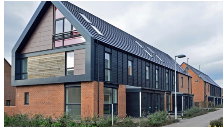
Commonwealth Games Village, Dalmarnock (Source: cruden-ltd.co.uk)
