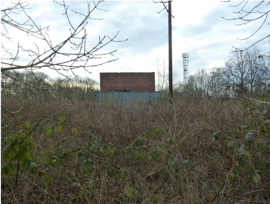
Photograph A: Roofless building.
