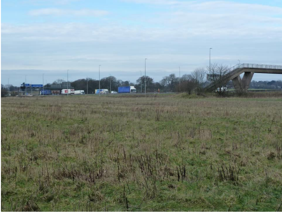
Photograph C: Showing one of the extensive and hazardous crossing points imposed by the M62.
