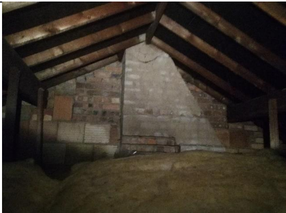
Photograph 29: Partion wall within 462 Poplars Avenue, shared with 460 Poplars Avenue
