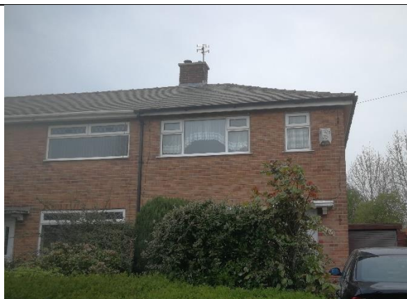
Photograph 12: General condition of 460 Poplars Avenue
