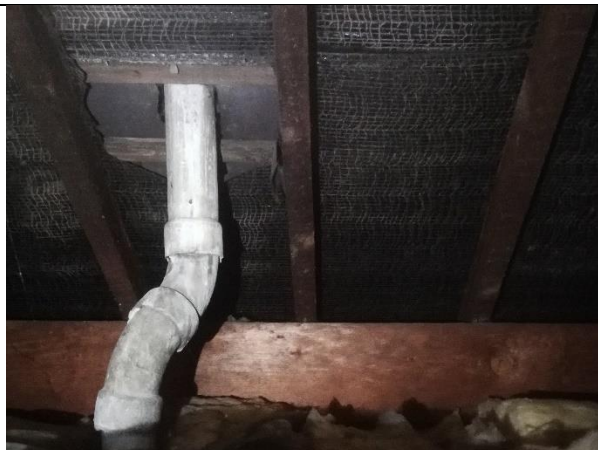
Photograph 31: Pipe going through slate to exterior (462 Poplars Avenue).
