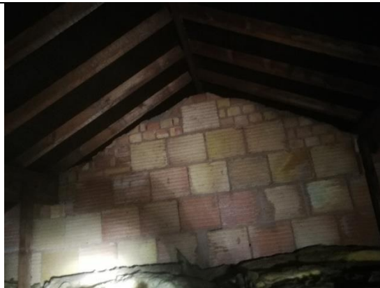
Photograph 30: Partion wall within 462 Poplars Avenue, shared with 464 Poplars Avenue. Large gap running along the top of the wall
