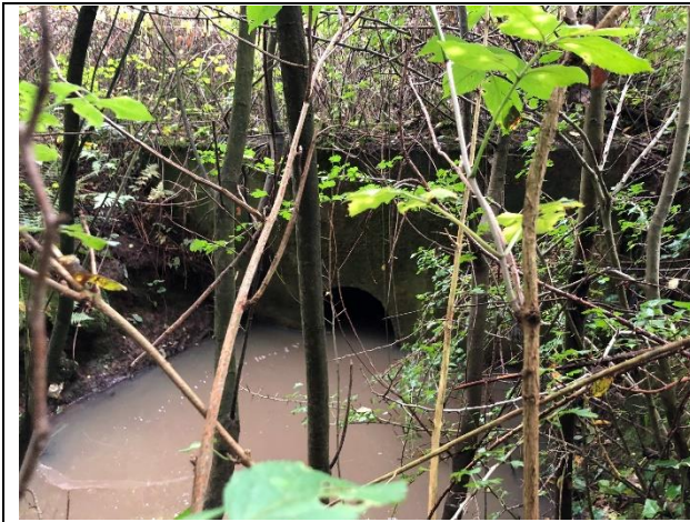
Photograph 85: Culvert within the very southern end of Spa Brook
