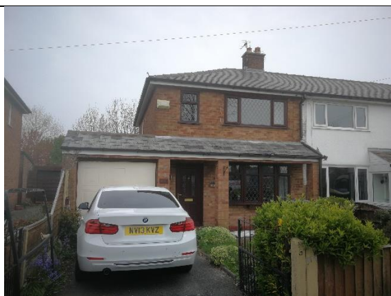
Photograph 9: Open porch with slate roof (458 Poplars Avenue)
