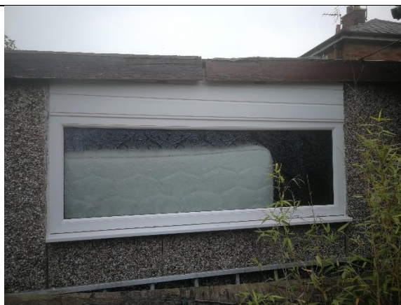
Photograph 47: PVC window on site of garage associated with 458 Poplars Avenue.
