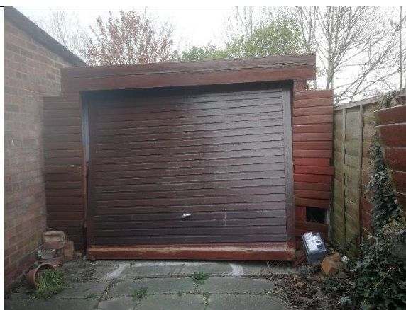
Photograph 45: Front of garage associated with 458 Poplars Avenue with wooden façade; door at an angle
