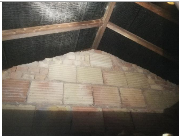
Photograph 33: Partition wall within the loft space of 464 Poplars Avenue, shared with 462. Large gap (10cm-30cm wide).
