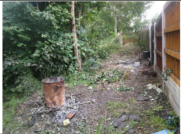
Photograph 25: Garden incinerator with fire damaged trees, Compartment C
