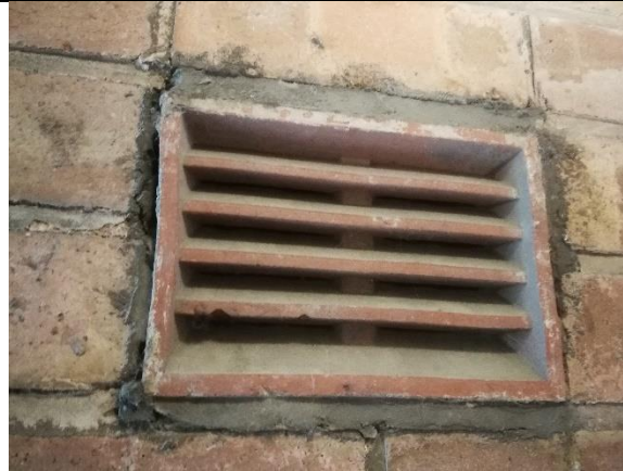
Photograph 55: Grilled vent in the side alley between 462 and 464
