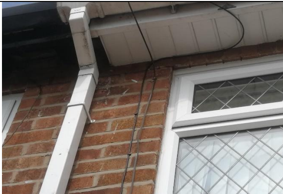
Photograph 17: Liming present at gap between white and black boxed soffits, indicating nesting birds (464 Poplars Avenue).
