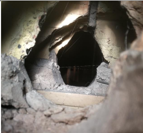
Photograph 25: Former pipe run in partition wall between 458 and 456 Poplars Avenue.
