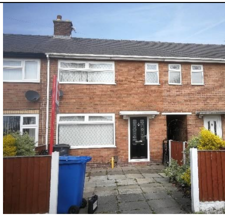
Photograph 16: General character of 464 Poplars Avenue
