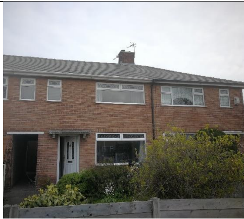
Photograph 14: General character of 462 Poplars Avenue
