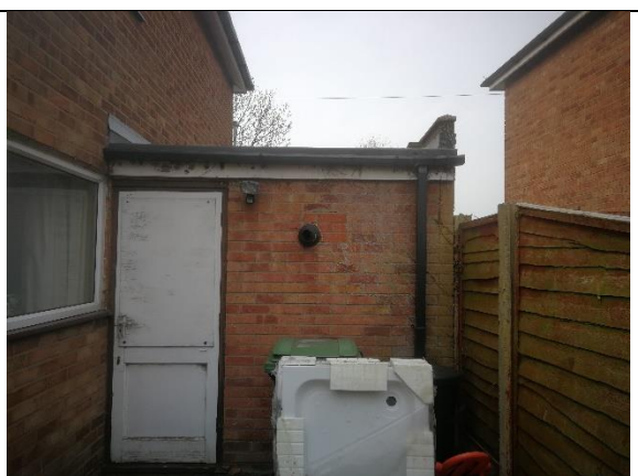
Photograph 40: Rear of garage outbuilding associated with 458 Poplars Avenue
