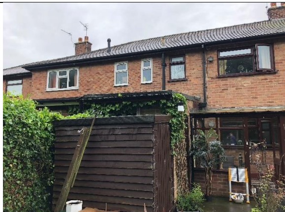
Photograph 36: Brick outbuilding and lean-to shed associated with 348 Poplars Avenue
