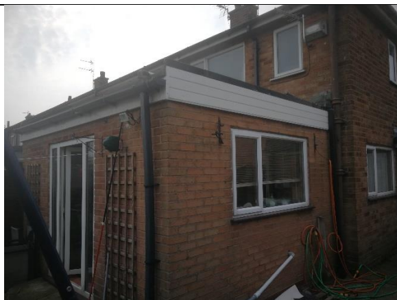
Photograph 11: Rear extension of 458 Poplars avenue with cladding and gutterboard
