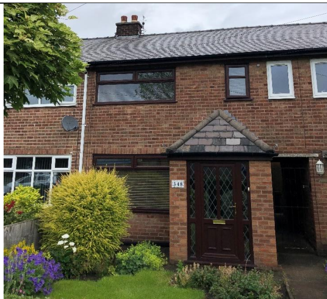
Photograph 6: Small porch present around front door, with slated roof (348 Poplars Avenue)
