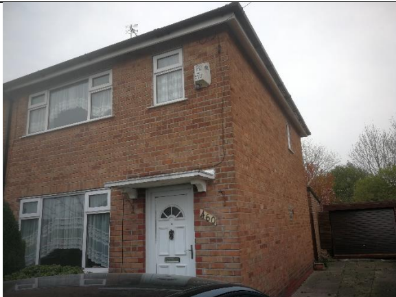
Photograph 13: Sloping boxed PVC soffits at 460 Poplars Avenue
