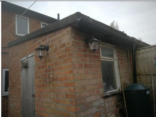
Photograph 48: Outbuilding contemporaneous with 462 Poplars Avenue
