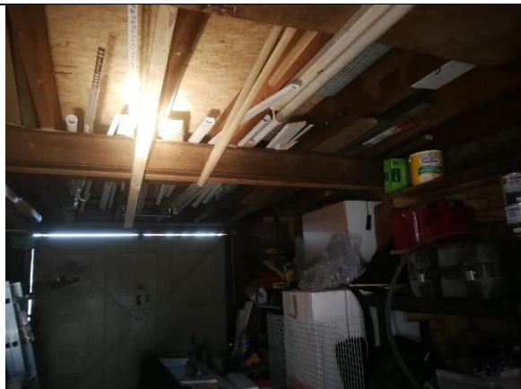
Photograph 42: Interior of garage associated with 458 Poplars Avenue
