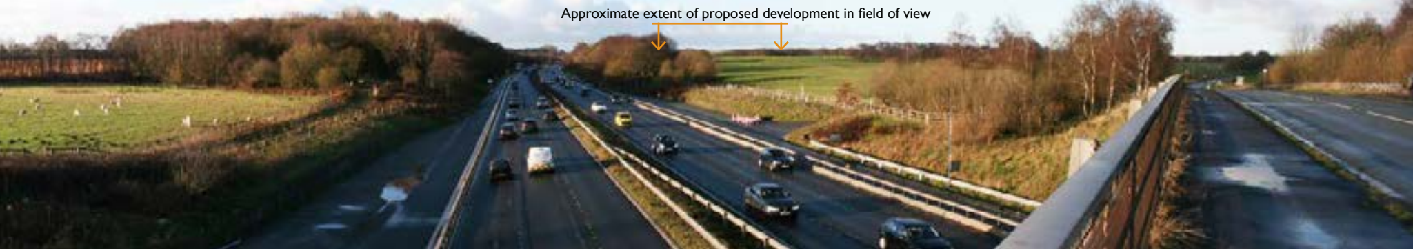
VP20 Looking west along M62 Motorway from B5212 Holcroft Lane motorway bridge towards Site
