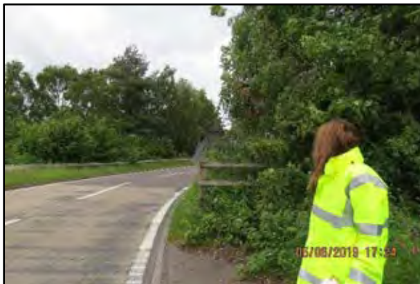
Restricted mutual visibility at the slip road
