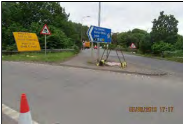
Existing footway at the slip road
