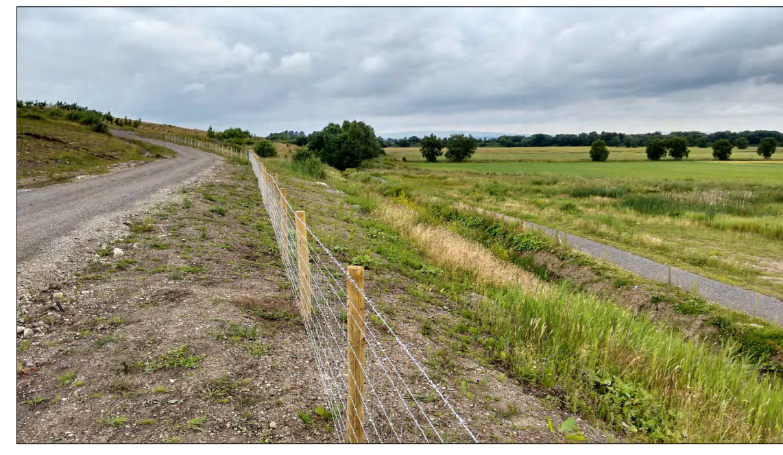
PHOTOGRAPH 5 : DITCH ALONG EASTERN SITE BOUNDARY WITH PUMPING CHAMBER FOR OUTFLOW
