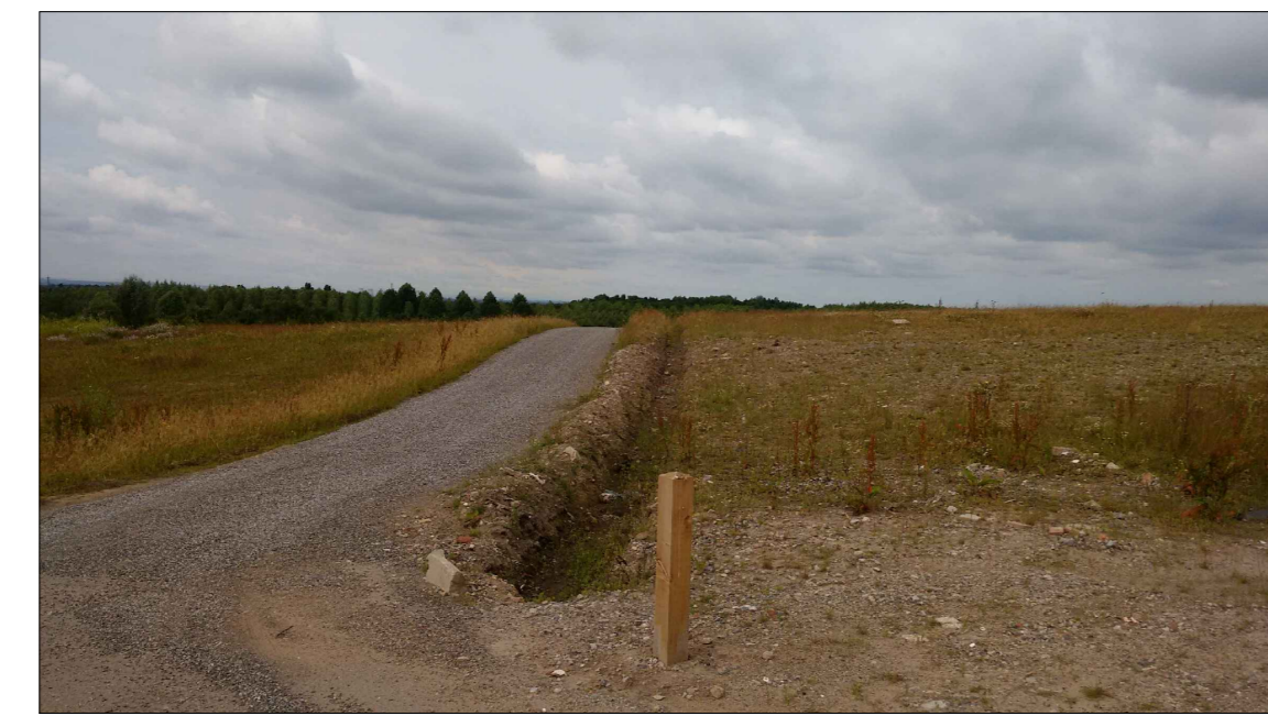
PHOTOGRAPH 7 : TYPICAL DITCH ARRANGEMENT ON CAPPED LANDFILL DOME
