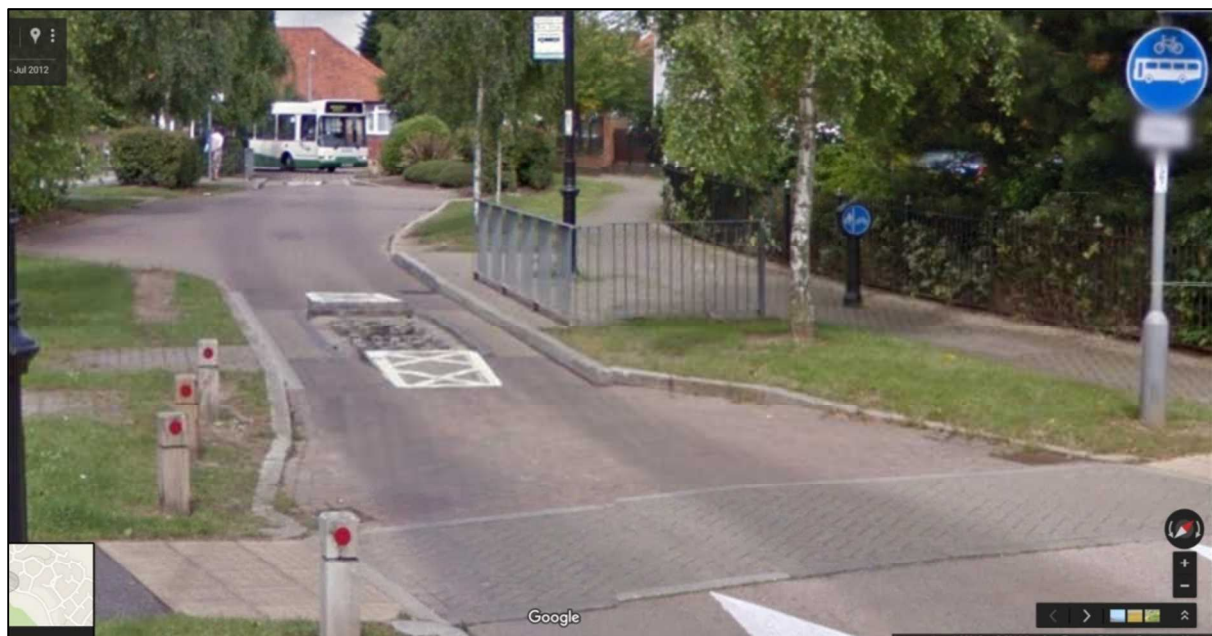
Figure 7.1 – Bus gate example (Ravenswood)
