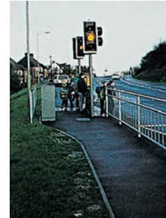
The introduction of guardrail may require footways to be improved to maintain adequate width.
