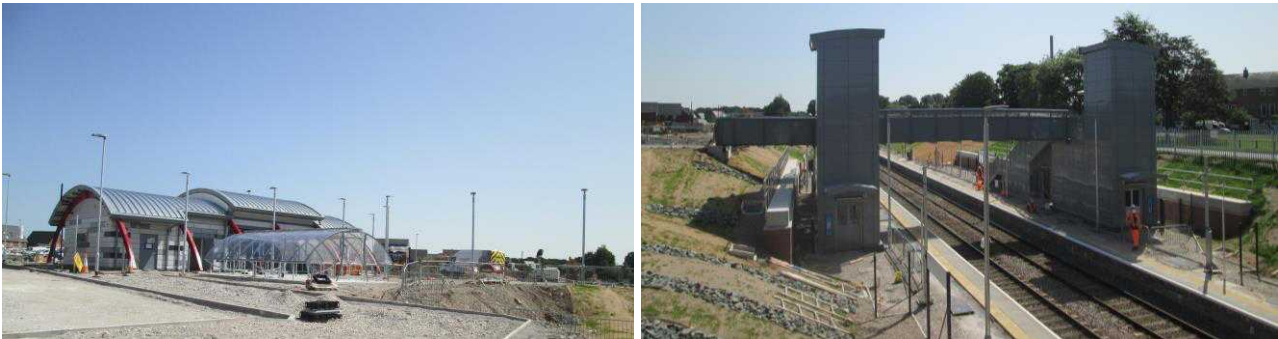
Figure 10.3 -Warrington West Station Construction Work
