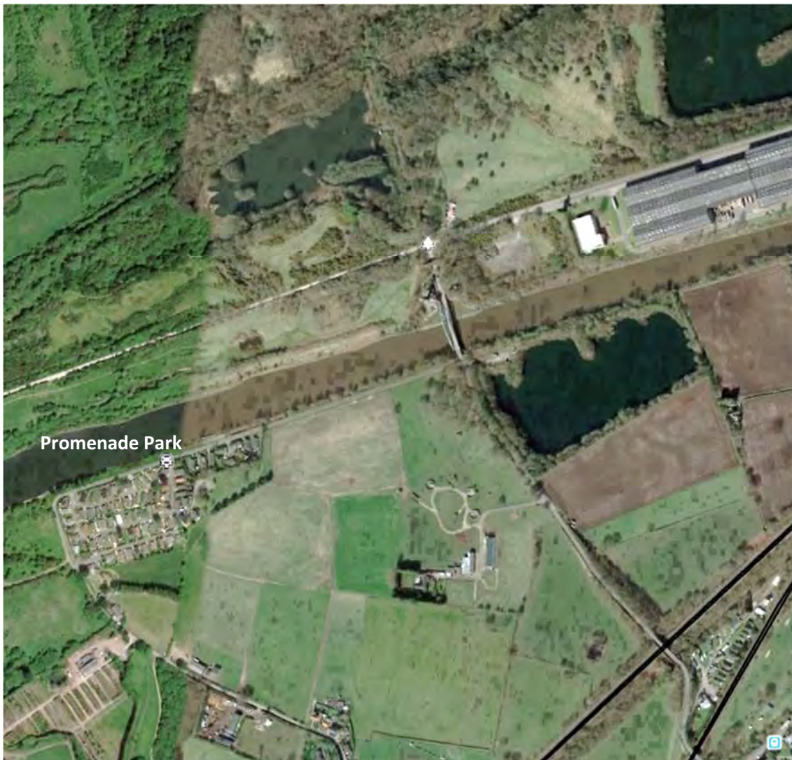
Figure 13: Aerial photograph of Promenade Park in relation to the Ship Canal
