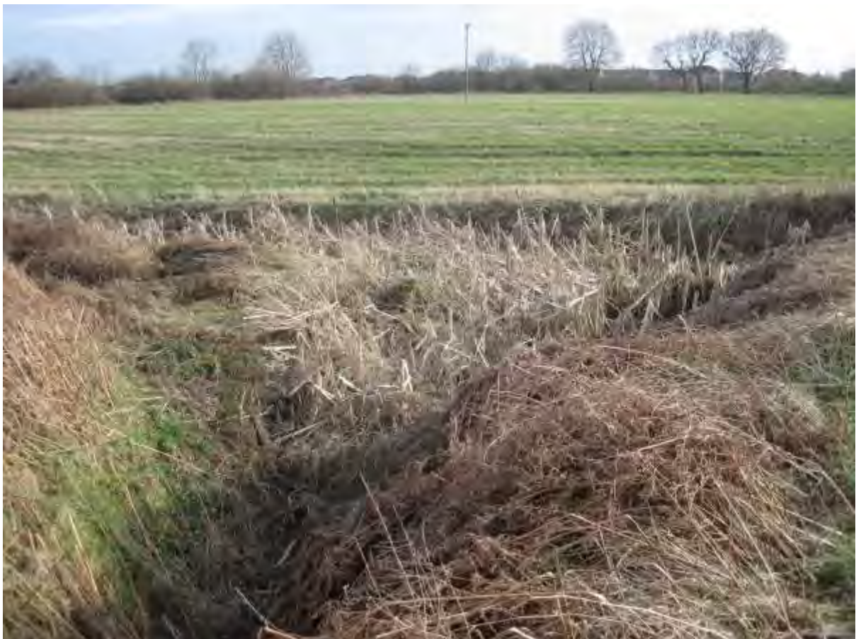
Photo 8 – Looking south at the attenuation basin, which was dry.
