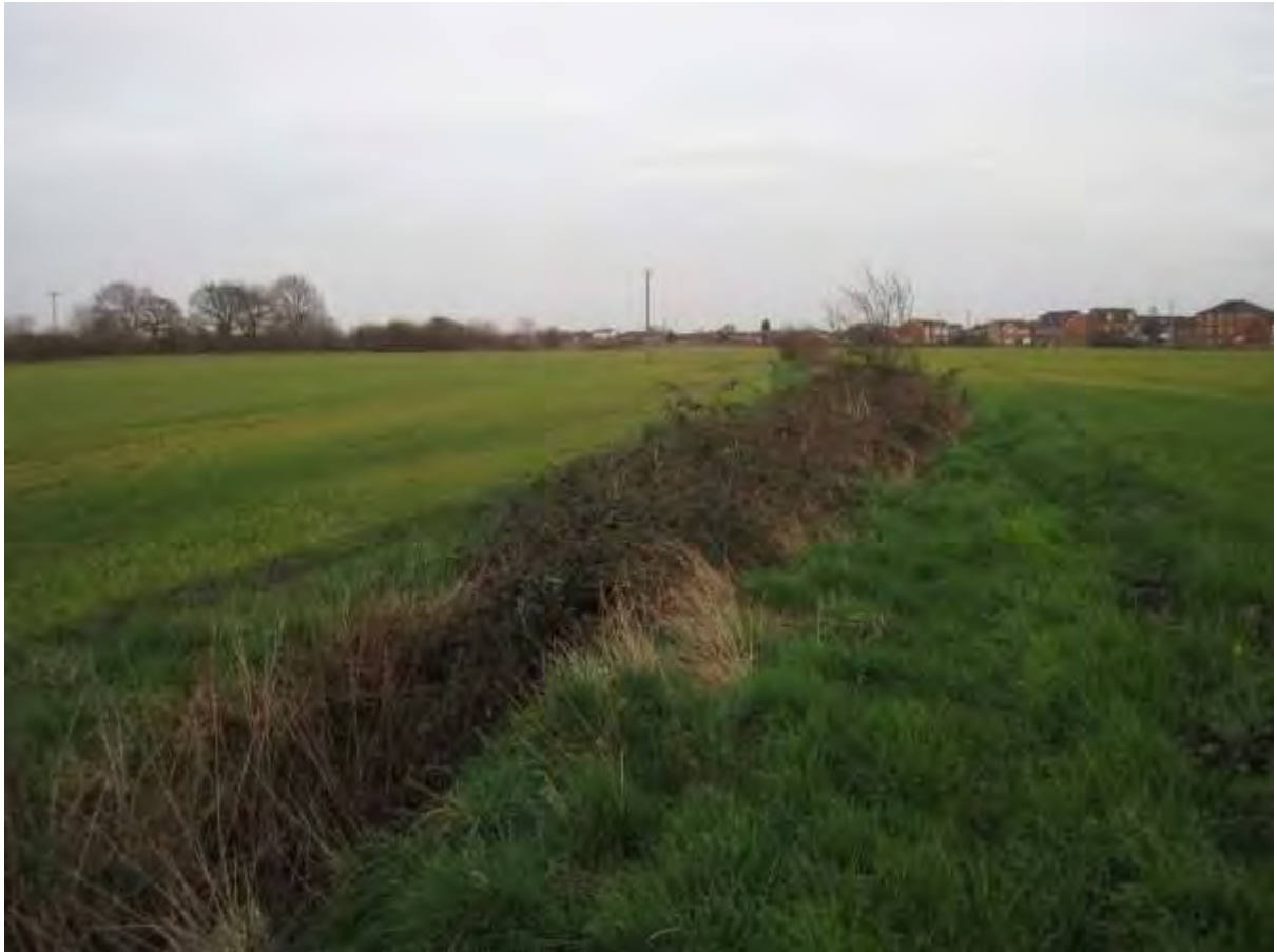
Photo 21 – Looking east at the ditch on the western site boundary.
