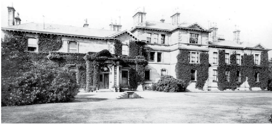
Historical photo of the front of Beechwood Manor
