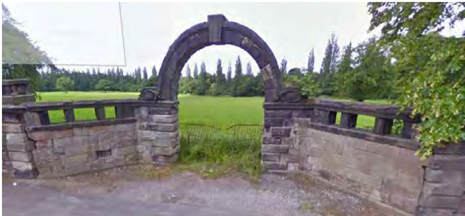
The existing archway into what would have been the entrance to the estate.
