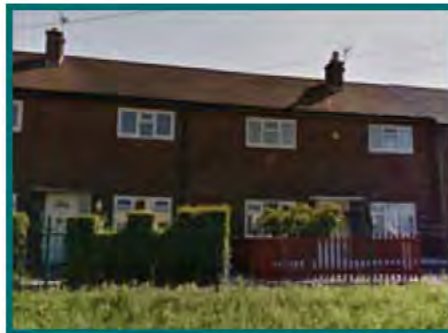
SOCIAL HOUSING A significant amount of post-war social housing was built in small estates to the southwest and south of Chapel Street.
