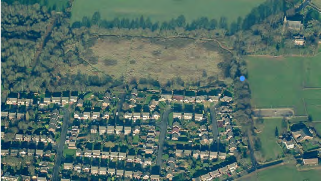
Bird's Eye view of the site from the south
