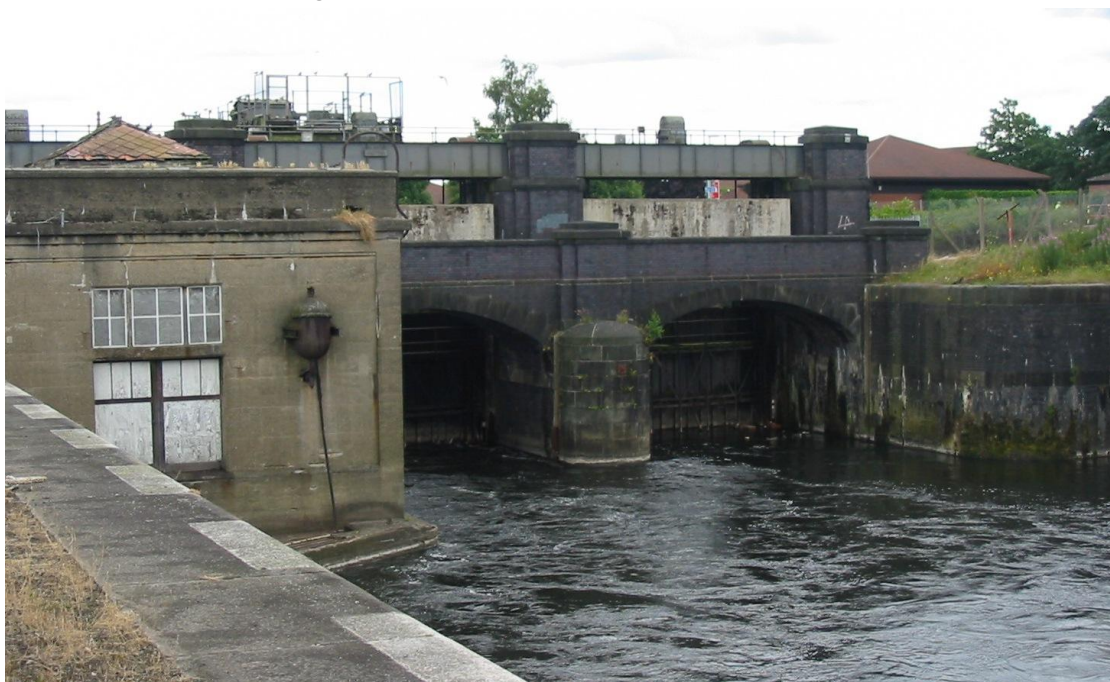
Figure 5-4: MSC Latchford Locks Sluice Gates
