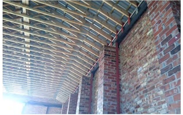
Photograph 2: Building open to trusses with no cavity walls
