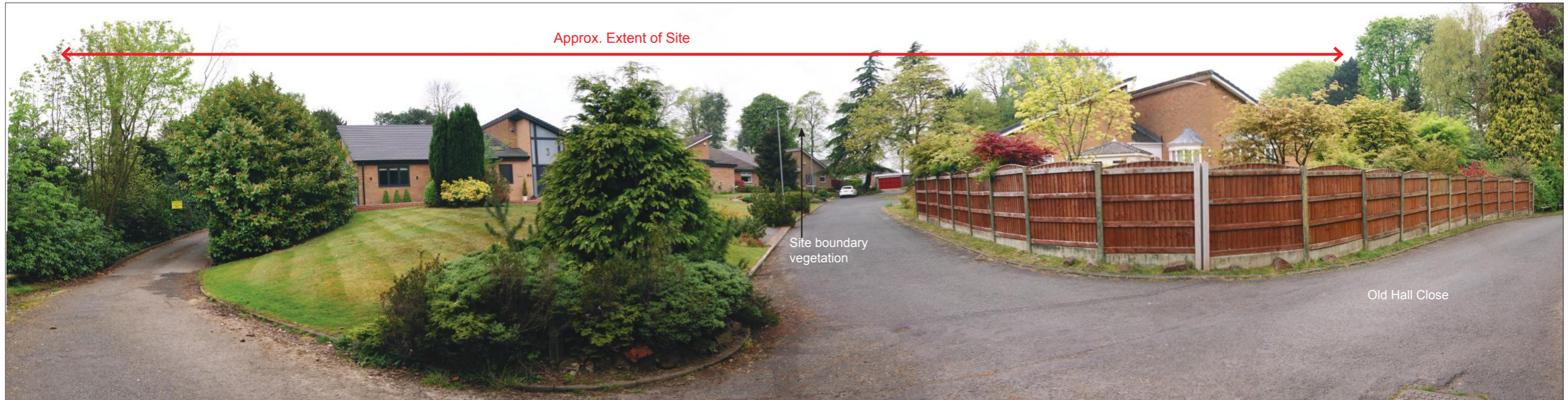
Photoviewpoint 3: Taken from Old Hall Close on the southern boundary on the site Distance from Site: 132m Orientation North-West Coordinates: X: 360497 Y: 385527
