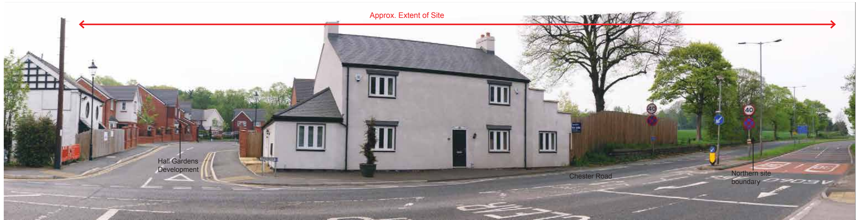
Photoviewpoint 1: Taken from Chester Road looking south towards the northern boundary of the site Distance from Site: 28m Orientation South Coordinates: X: 360352 Y: 385958
