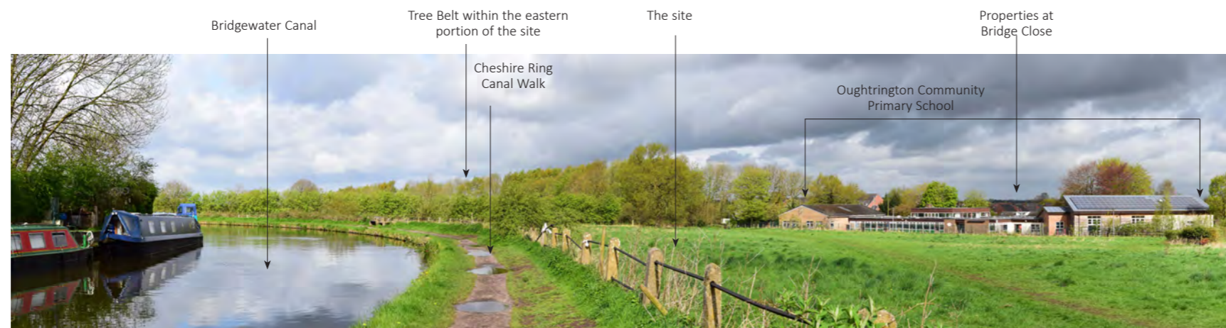
Photo 4.1 - View from the Cheshire Ring Canal Walk looking west.
