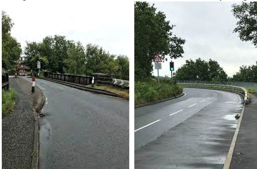
Figure 9. Moore lane where it crosses the railway bridges
