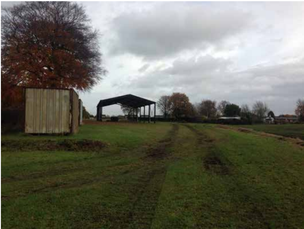
7. View looking eastwards towards existing agricultural buildings.
