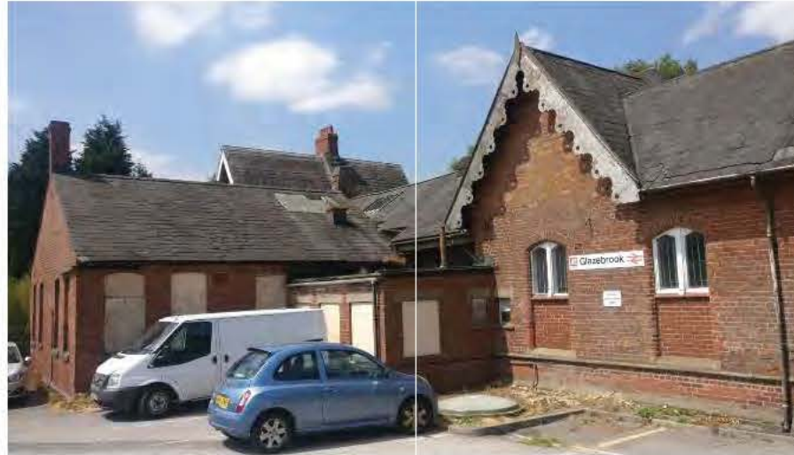
Glazebrook rail station concourse
