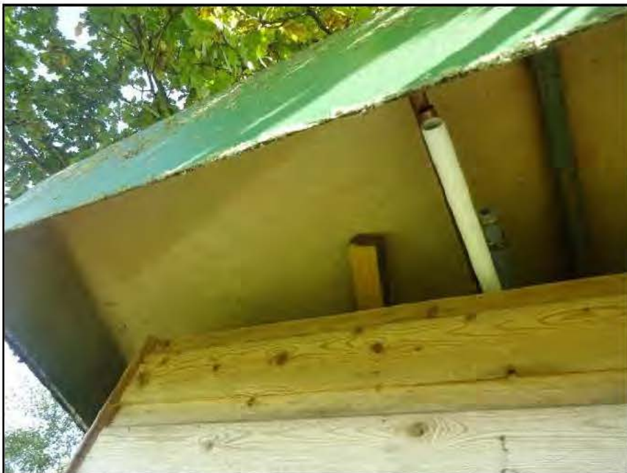
Photograph 9 showing the roof
