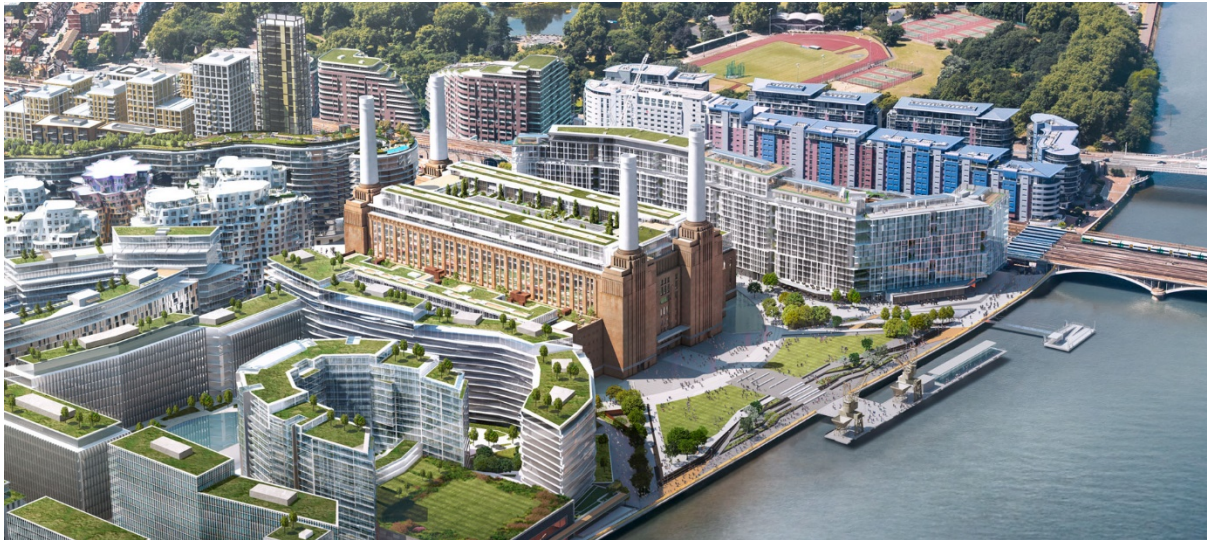
Figure 1: Successful conversion of Battersea Power Station, London provided 4,239 homes onto the 39 acre site, alongside shopping outlets and other attractions / amenities.
