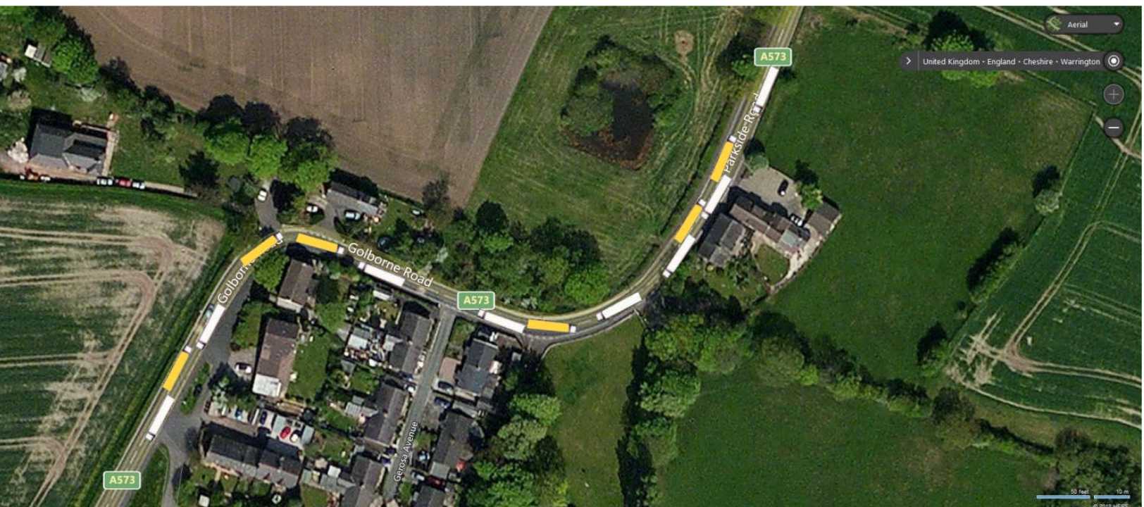
Schematic view of congestion grid-lock at the Hermitage Green “S” Bend on Golborne Road/Parkside Road if the Proposed Parkside Link Road goes ahead.
