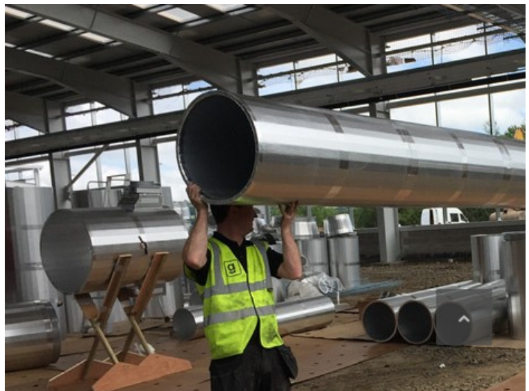
Figure 18: Example of alternative ductwork
