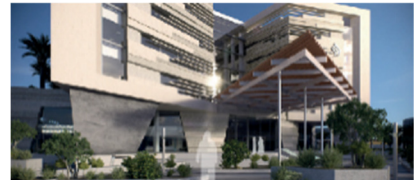
Data Centre Infrastructure Management (DCIM)
