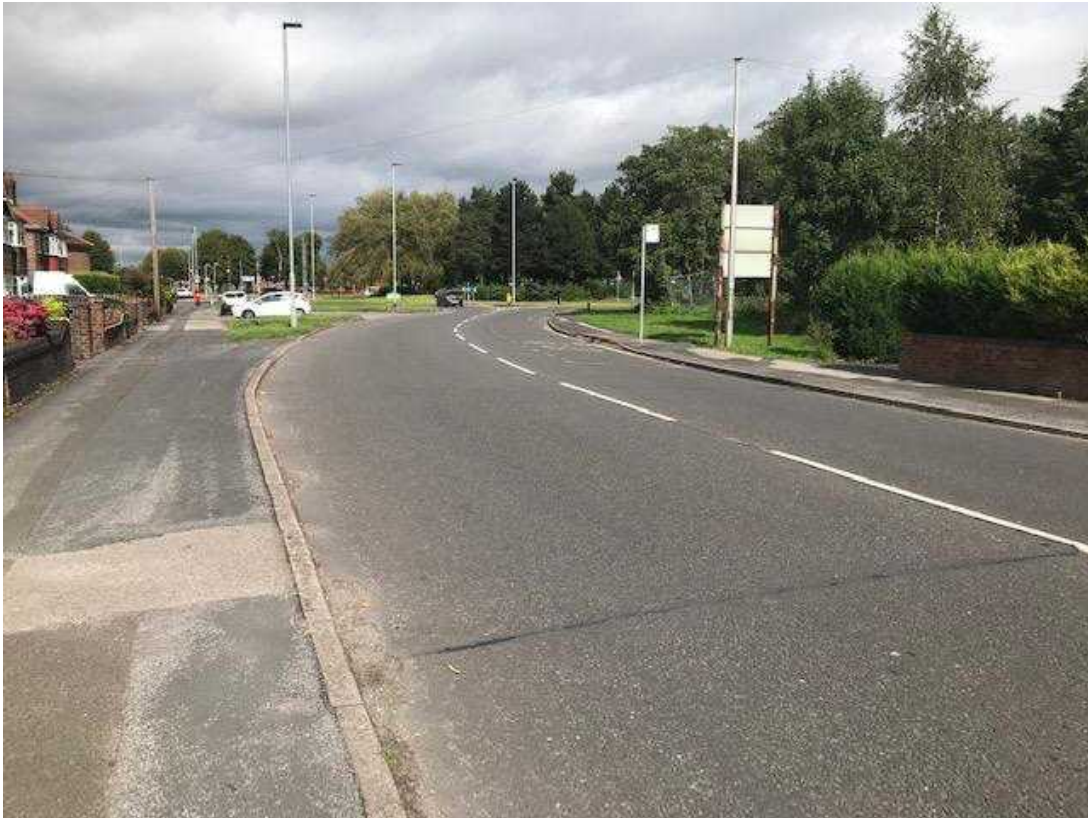
Orford Road approach to roundabout
