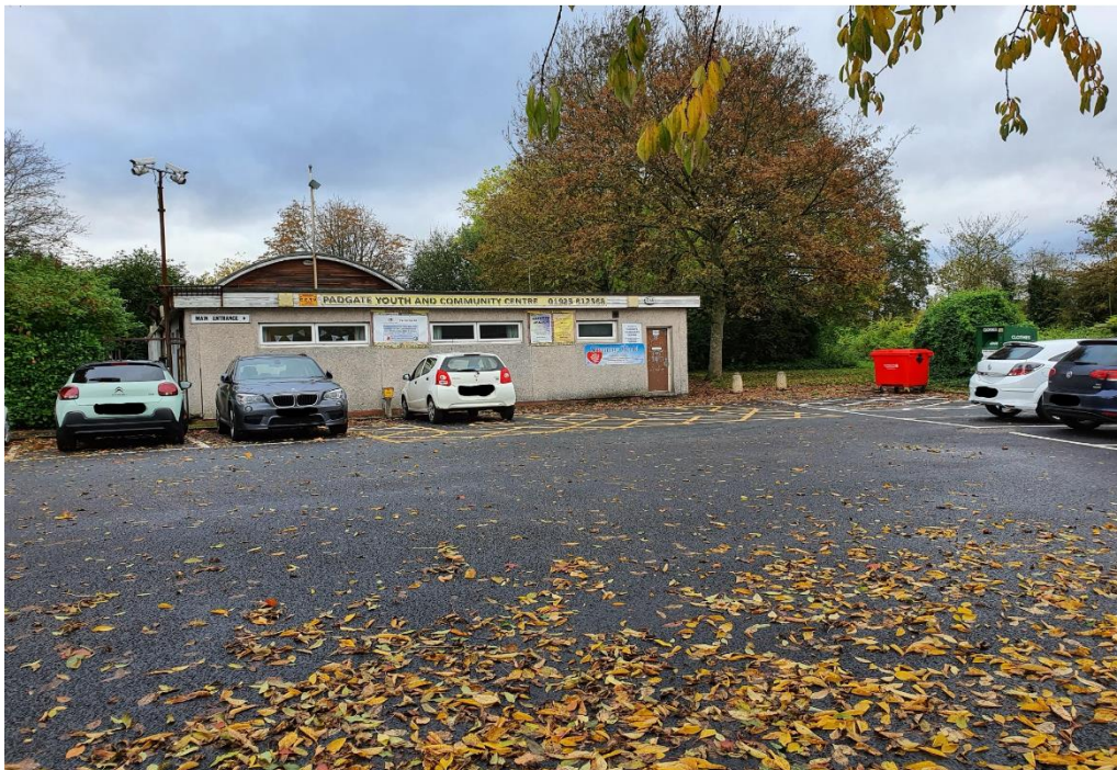
Figure 6 - Padgate Youth & Community Centre
