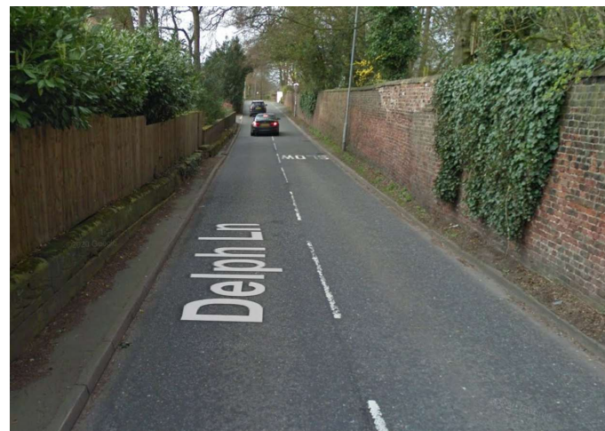
Narrow and poorly lit road
