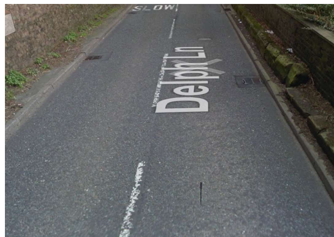
Combination of narrow road, lack of pavements and proximity to walls is dangerous for motorists, pedestrians and cyclists.
