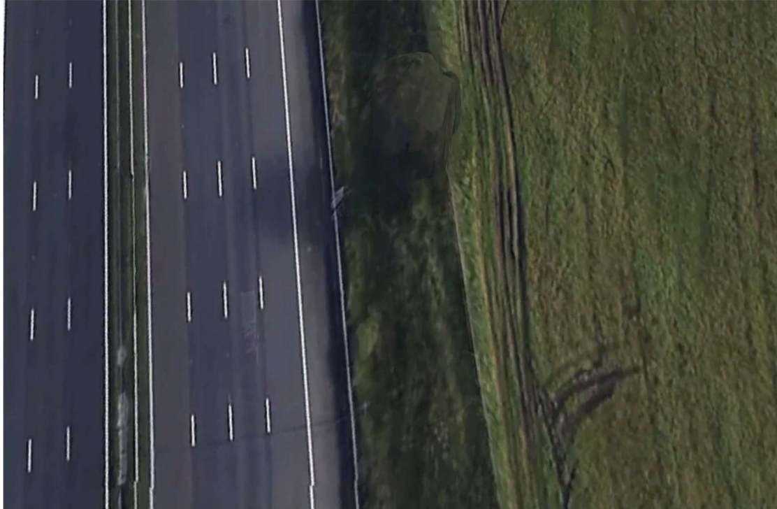
MP04 - 16 metres from highway
