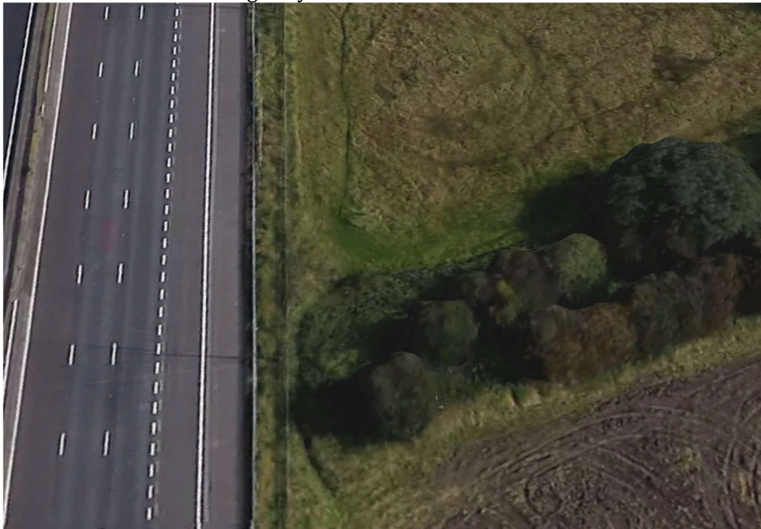
Embankment height = 1 metre below highway
