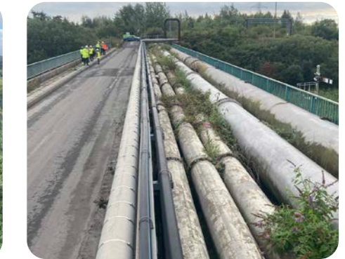
Photo of Fiddler's Ferry railway bridge
