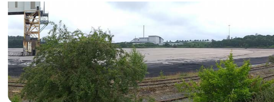
Photo of the coal pad
