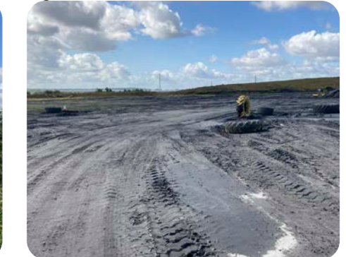
Photo of the ash lagoon currently under extraction
