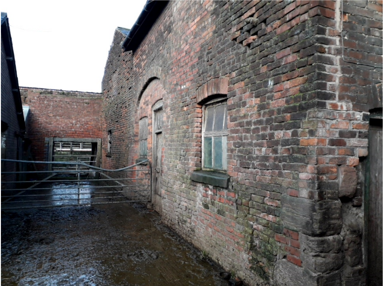
Figure 5: View from inner courtyard
