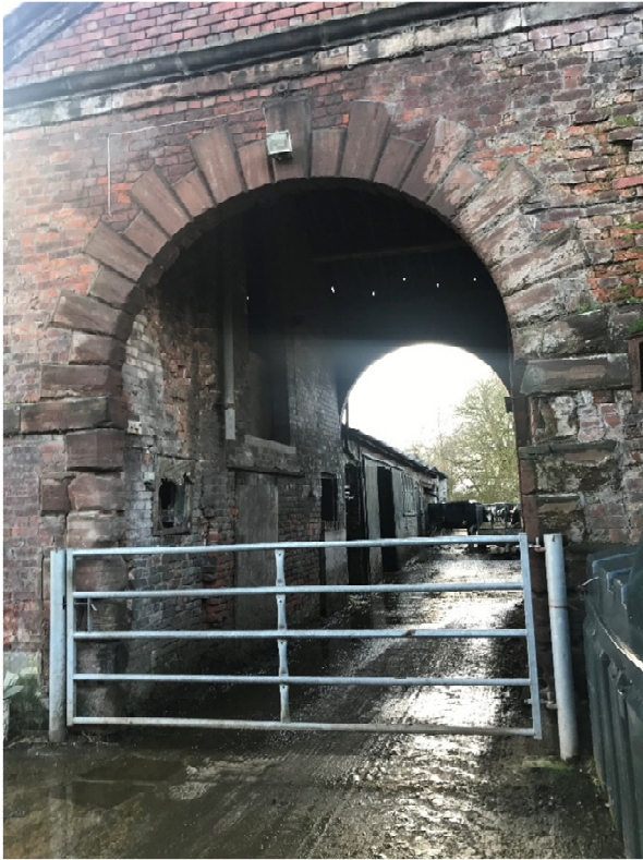
Figure 1: View to central arch of barn
