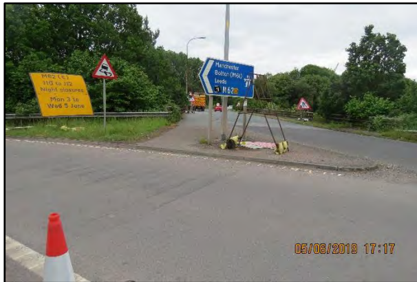
Existing footway at the slip road
