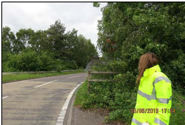
Restricted mutual visibility at the slip road
