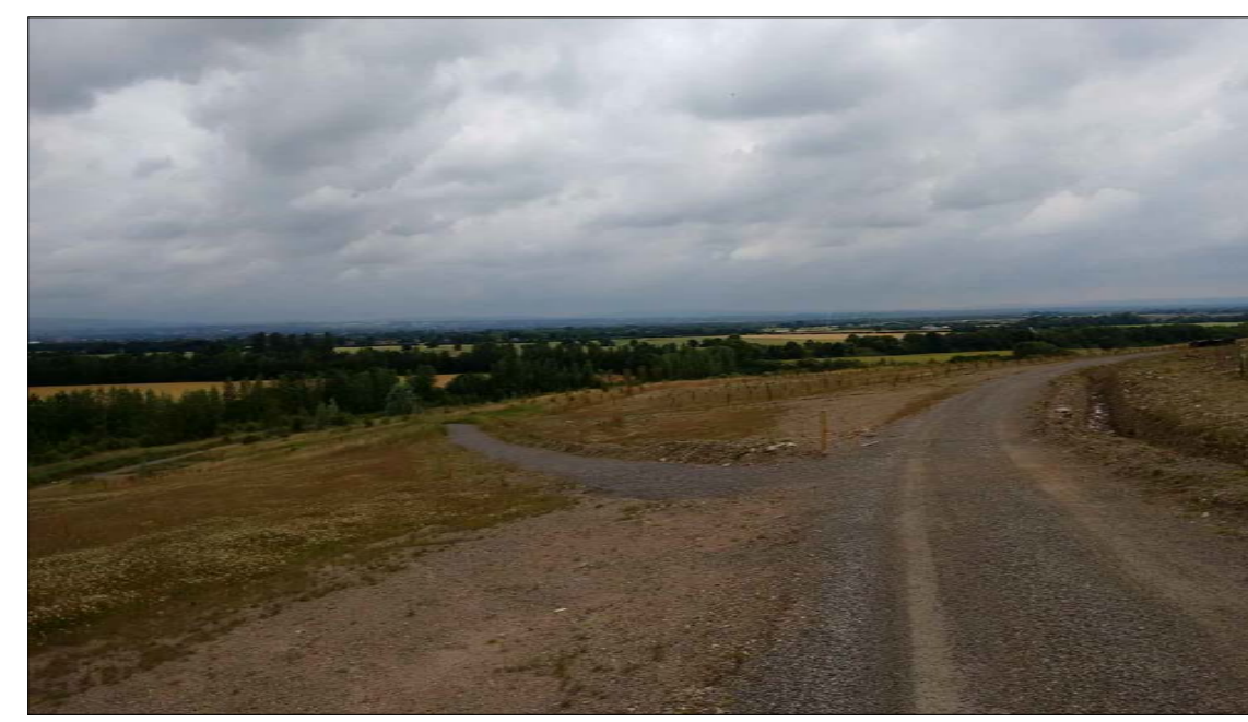
PHOTOGRAPH 14 : VIEW OF TRACKSIDE DITCH UP-GRADIENT OF ROAD WITH INSUFFICIENT FALL
