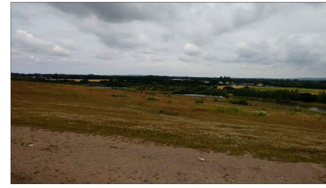
PHOTOGRAPH 8 : VIEW OF PONDS 1, 2 AND 4 FROM CAPPED LANDFILL
