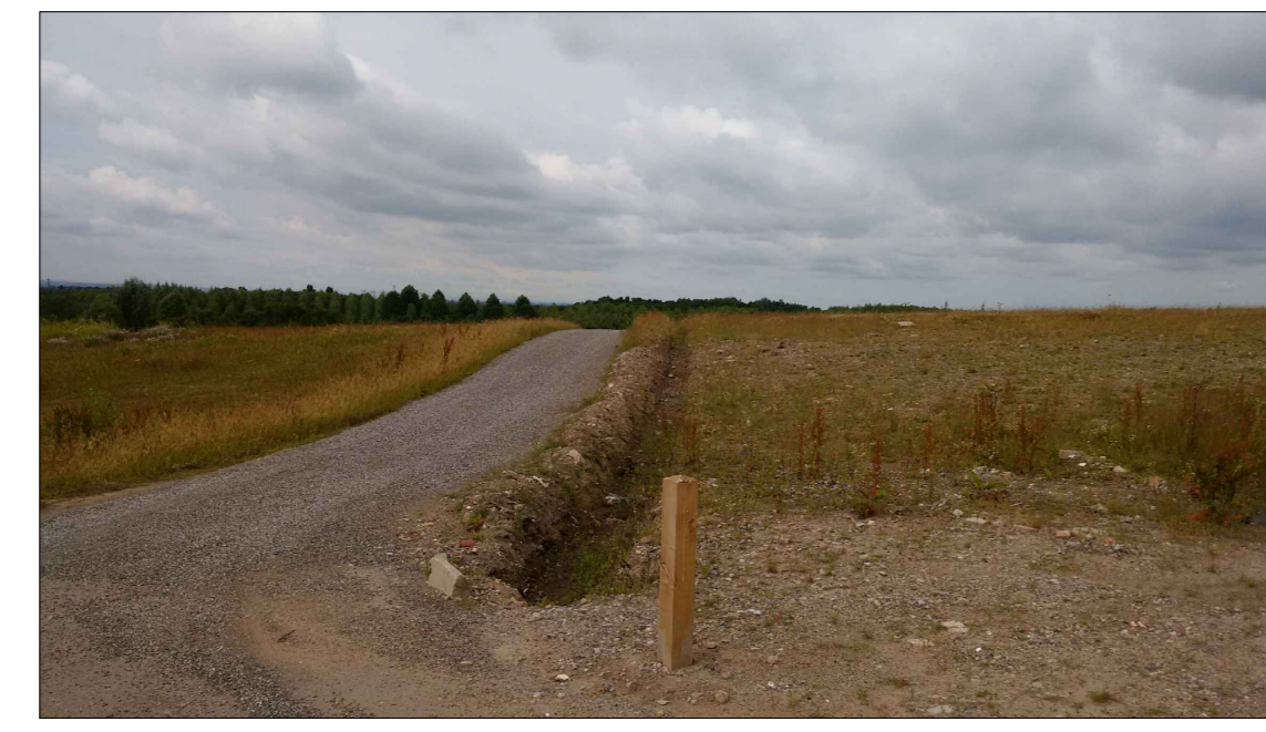
PHOTOGRAPH 7 : TYPICAL DITCH ARRANGEMENT ON CAPPED LANDFILL DOME
