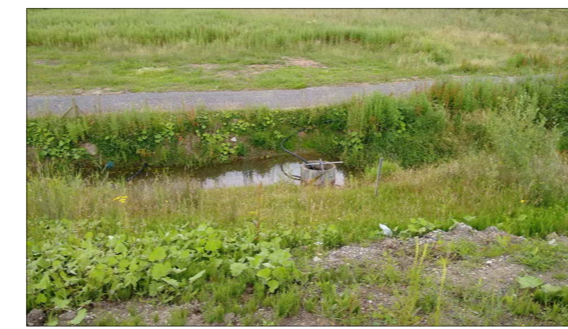
PHOTOGRAPH 12 : PUMPING CHAMBER IN DITCH ALONG EASTERN SITE BOUNDARY
