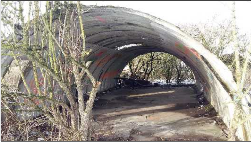
Plate 13: Disused corrugated iron sheds.
