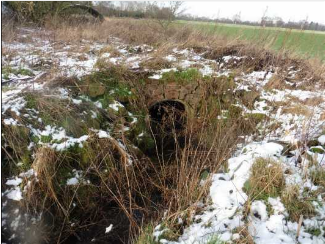
Plate 11: Brick-built culvert, possibly 20 th century.
