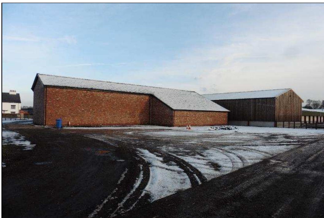
Plate 7: Large agricultural outbuildings to the south-east of Holcroft Hall
