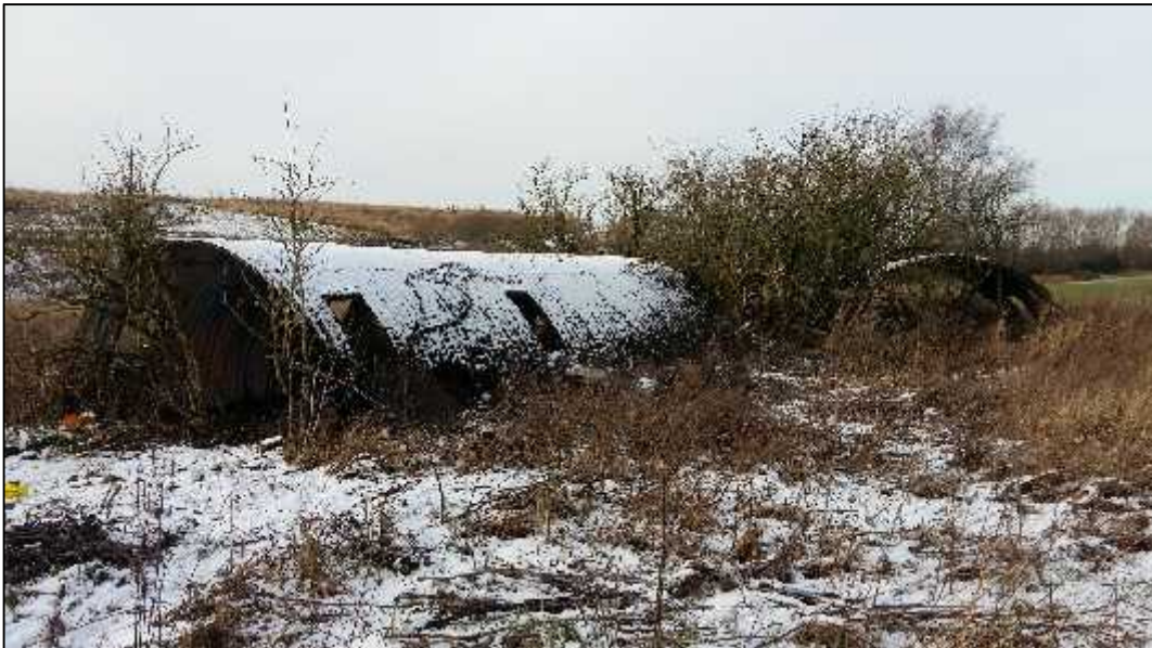
Plate 12: Disused corrugated iron sheds.
