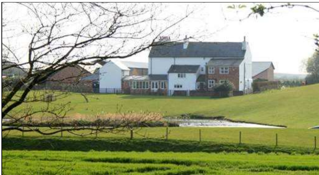
Plate 6: Rear elevation of Holcroft Hall
